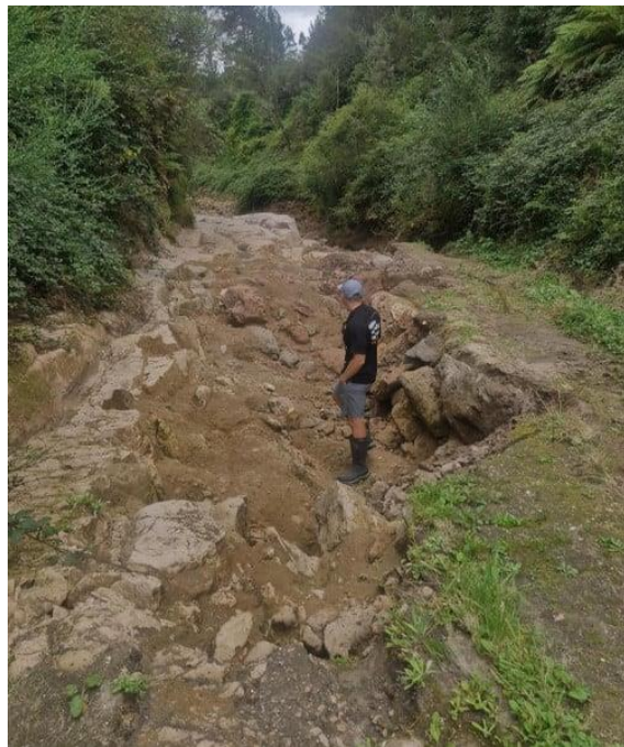
Some of the significant damage on the previously 4x4 track to the Waipapa River.
